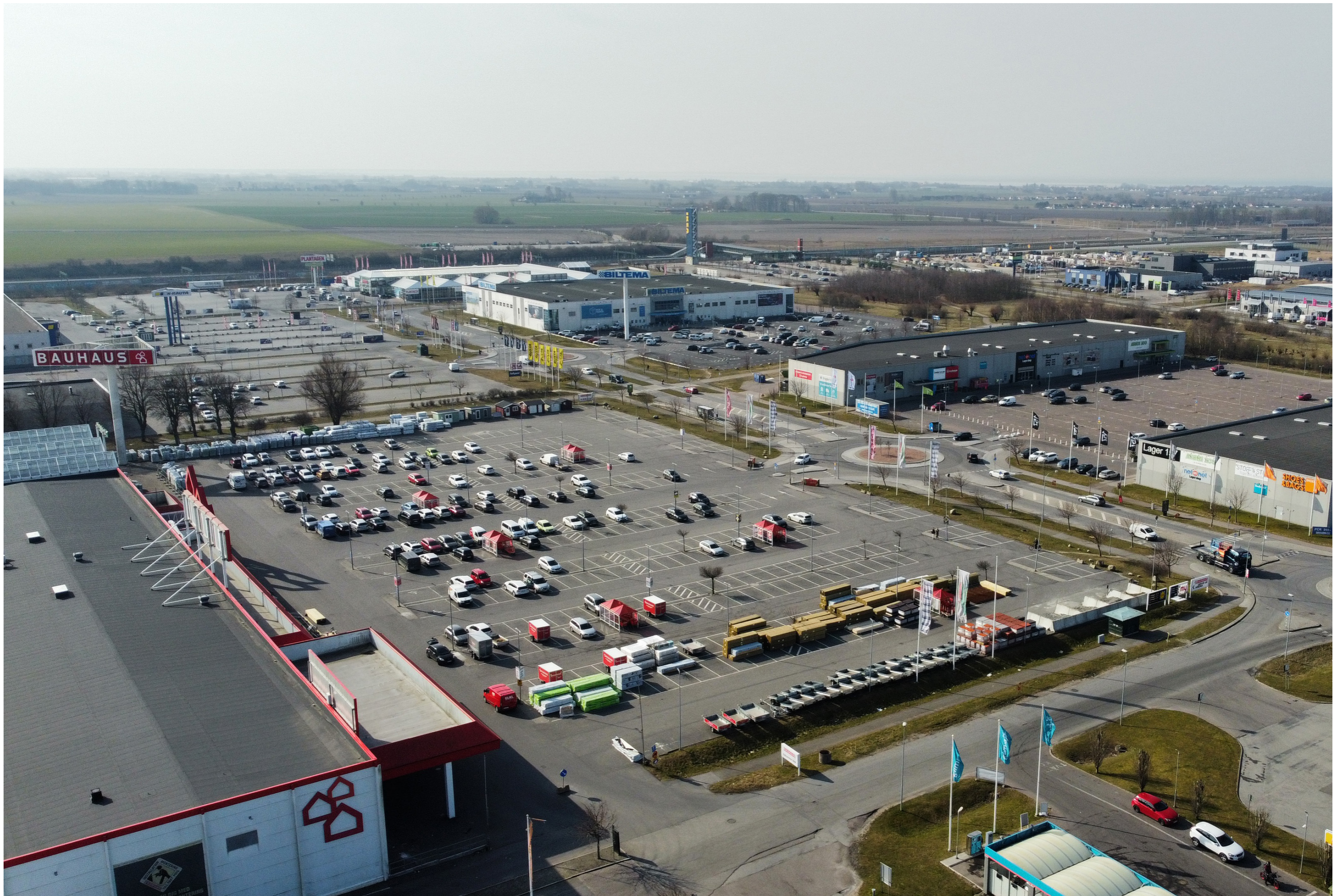
Figure 08: Drone footage of Svågertorp, the thesis project site.
