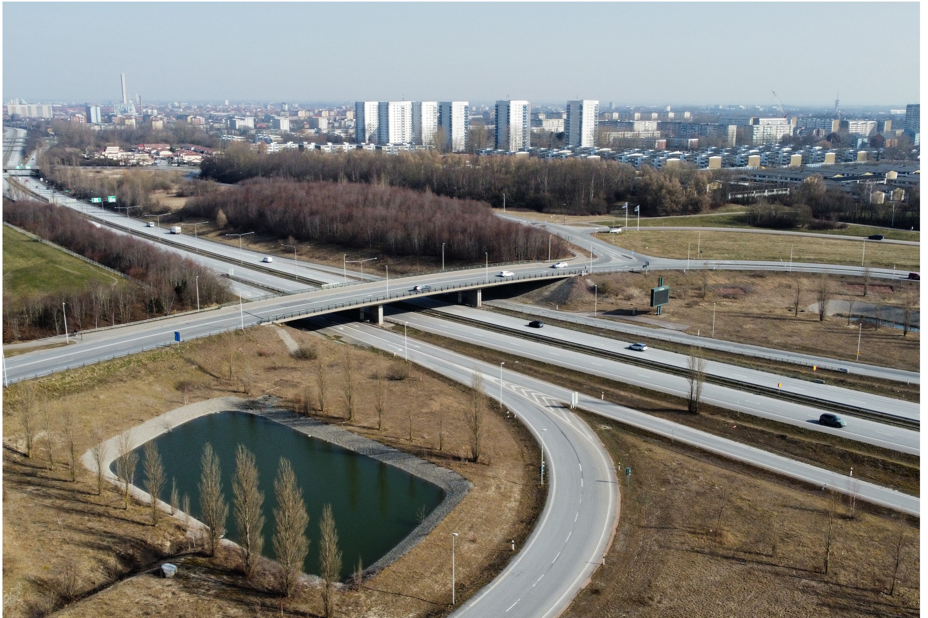
Figure 17: Drone footage of Svågertorp, the thesis project site.
