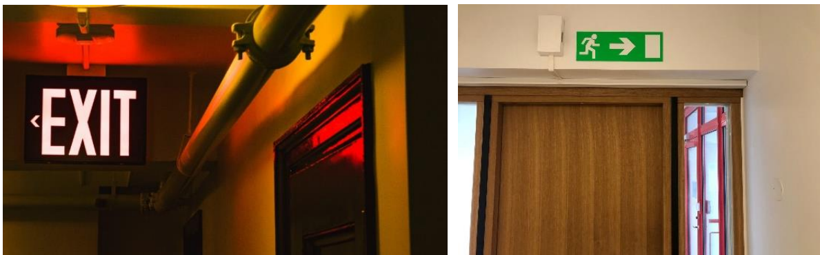
Figure 1: Left: Red Exit sign (2018, October 5). [Photograph]. Connected Fire. https://connectedfire.com/index.php/blog/2018/10/05/emergency-lighting-and-exit-signs , Right: ISO Exit Sign (Source: Author)
