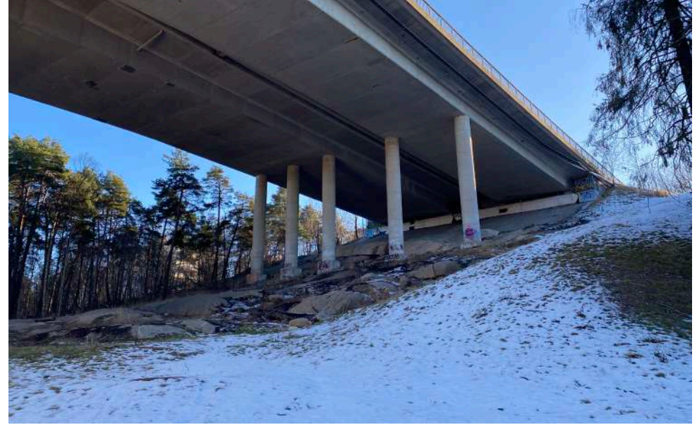
Figure 45. a slope under the bridge
