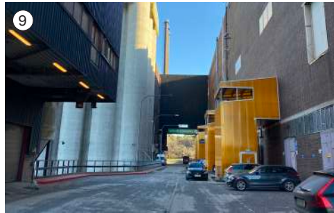
Figure 64. path between the brewery and silos
