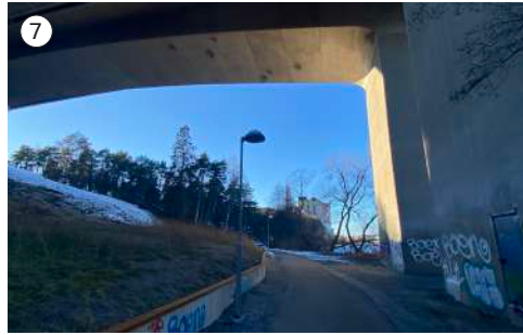
Figure 62. the path under the bridge
