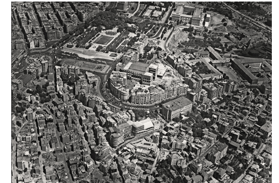
1.6 Aerial view of Taksim in the late 1950s.
