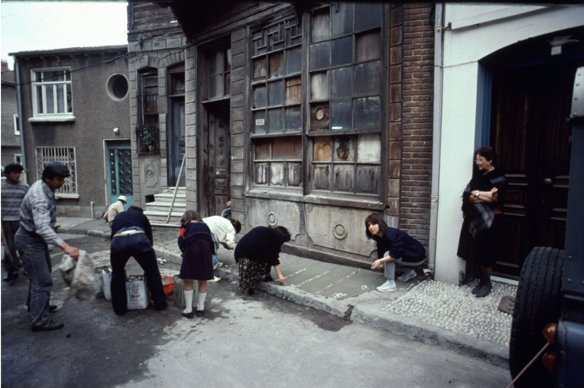
Figure 4 The people of Kuzguncuk are laying pebbles on the sidewalks with the architect, Cengiz Bektaş.
