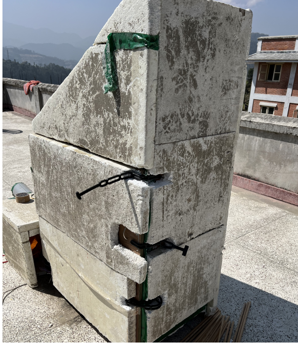
Figure 5: Exterior of rooftop dryer with new rubber strap installation
