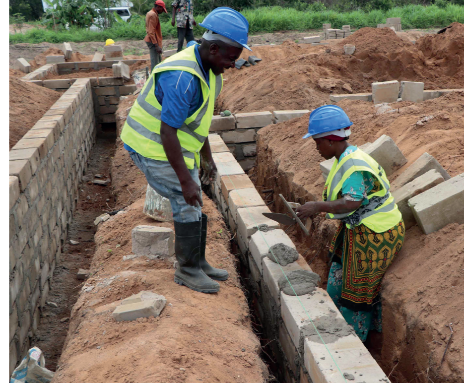
Fig. 15: Foundation and Wall Construction, image was taken by TAWAH
