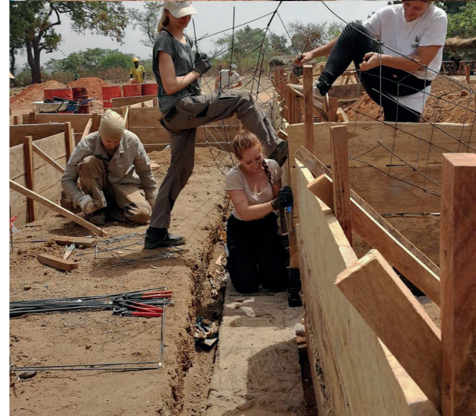
Fig. 16: Concrete Foundation picture taken by Julia Kasparek
