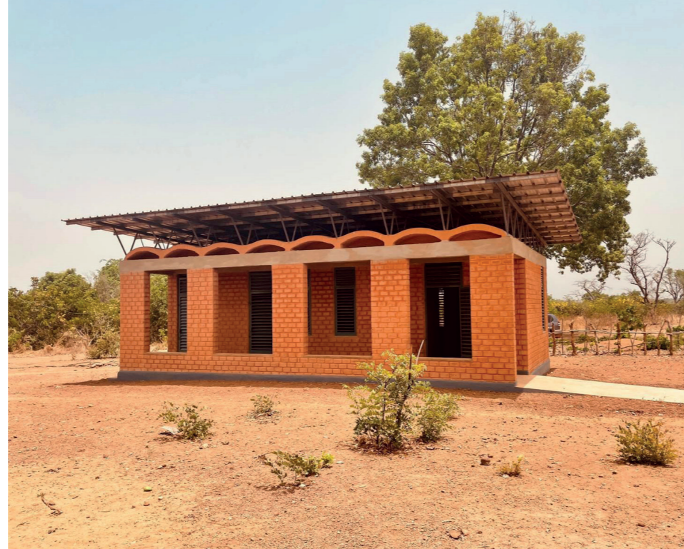
Fig. 21: Sanitation facility for a school project Guinea, RWTH Aachen (RWTH-Aachen, 2022)
