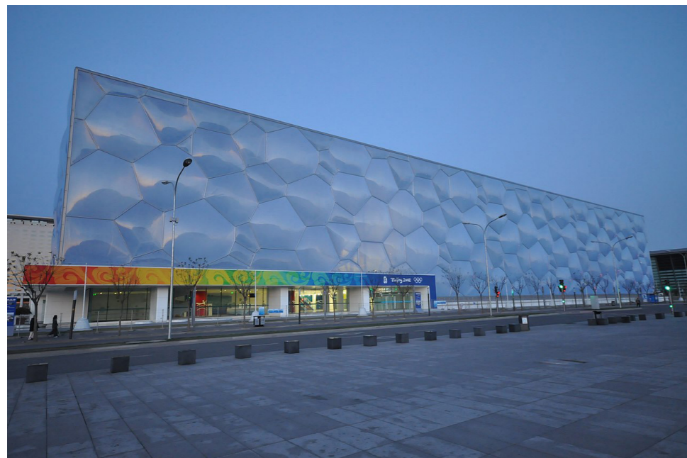
It could be argued that much of the contemporary architectural ornament stays on the surface of the building, rather than becoming three dimensional, like the projecting sculptural elements of traditional ornament (Picon, 2016). Water Cube (Lascar 2014)
