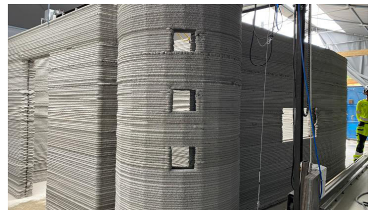
3D-printing (Heidelberg Cement n.d.)
