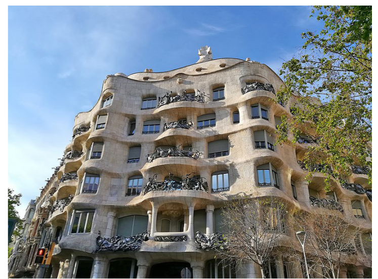
This design has some parallels to Casa Mila, by architect Antoni Gaudi. Its facade is also free-standing, which was very modern for its time. It also has elements of re-use, with the balconies having recycled scrap metal as its material. (Enric 2021)
