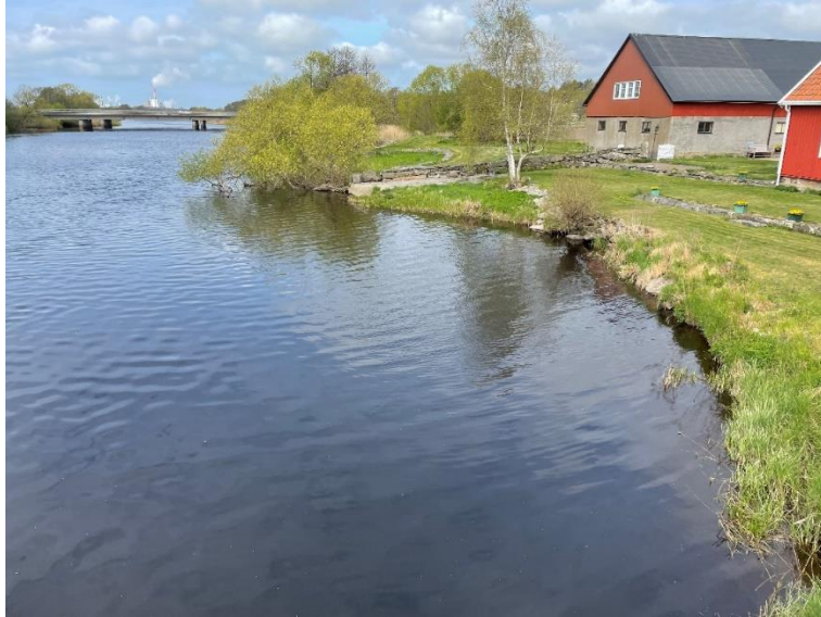
Figure 13. One of typical erosion problems at Viskan at downstream
