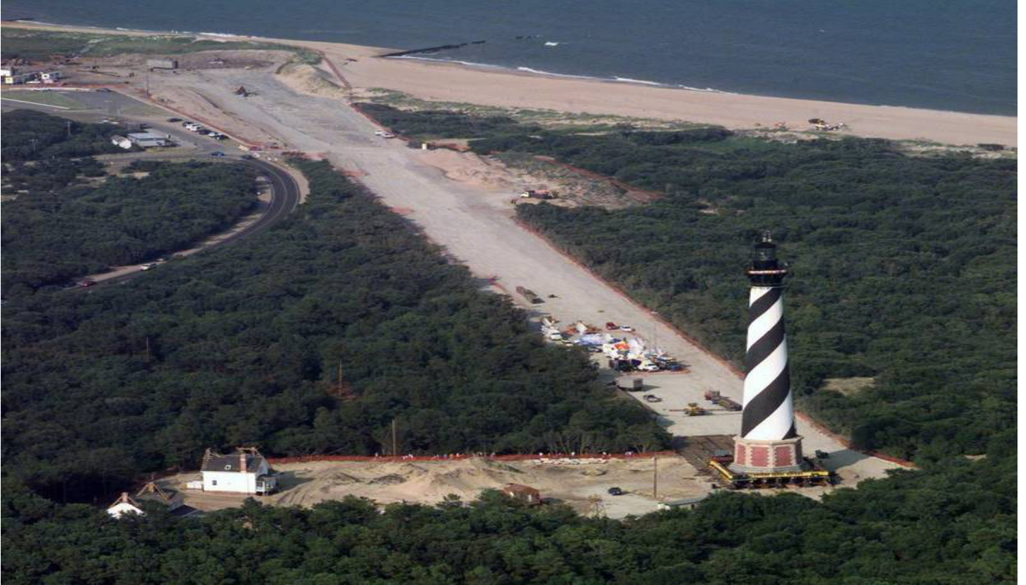
Cape Hatteras Lighthouse being moved 1 km inland in 1999. Image credit: DREW C. WILSON
