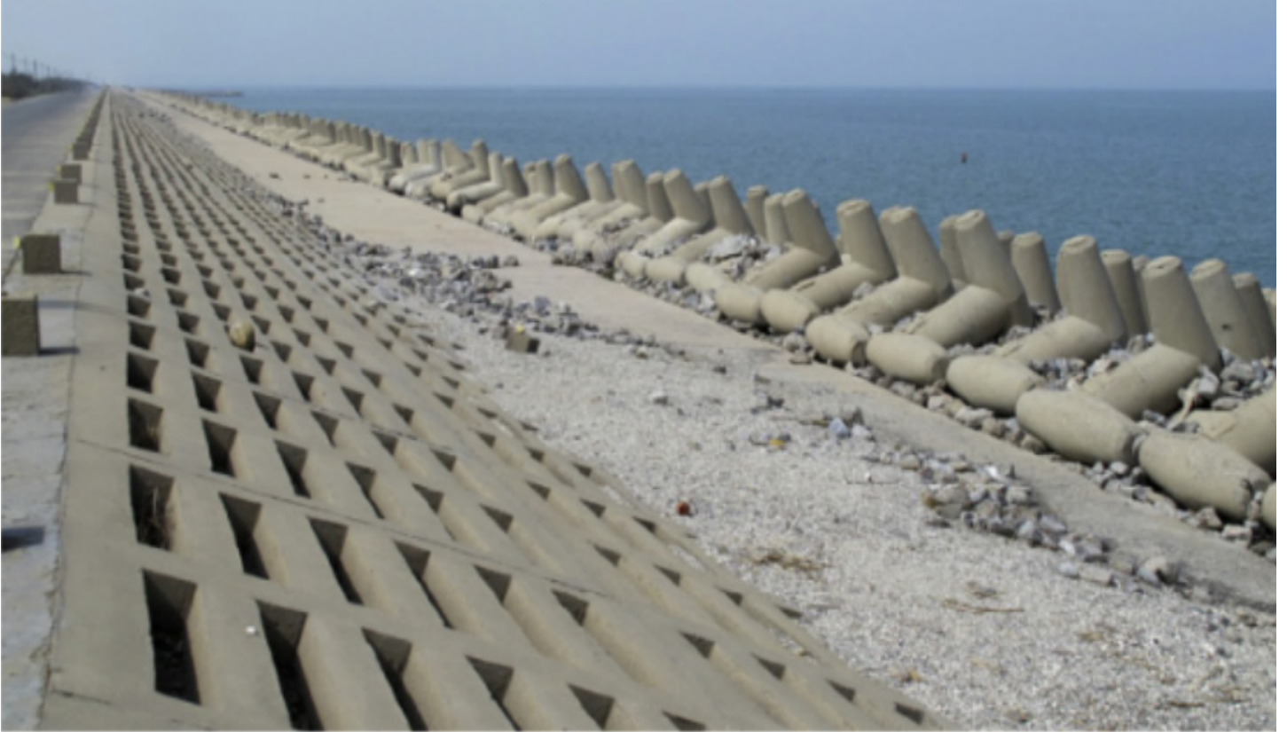
Sea wall in Gudong, Yellow river delta, China. Built in 1985 and named the ‘Coastal Great wall.’ Image credit: Williams, Rangel-Buitrago, Pranzini, Anfuso, 2018
