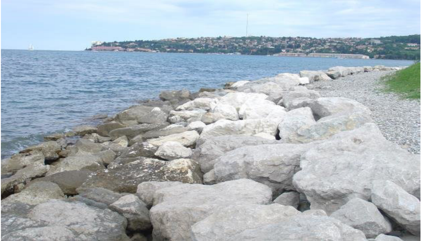
Revetments rock armor structure protecting a beach from erosion. (Čehovin & Zagar 2019)
