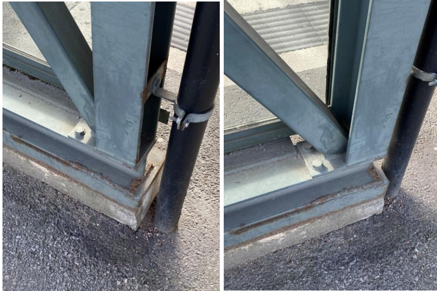
Figure 19: Two joined I-beams with a hollow square section beam (Photo: Daniel Rundström).
