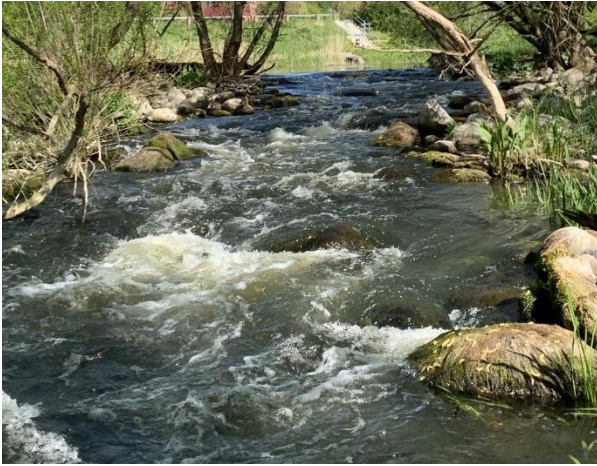
Figure 4. Upstream entry of the fishway, flow depth in pools is approximately 40-50 cm at the time of the visit.
