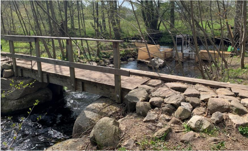
Figure 41. Upstream view over bridge and fishway entry
