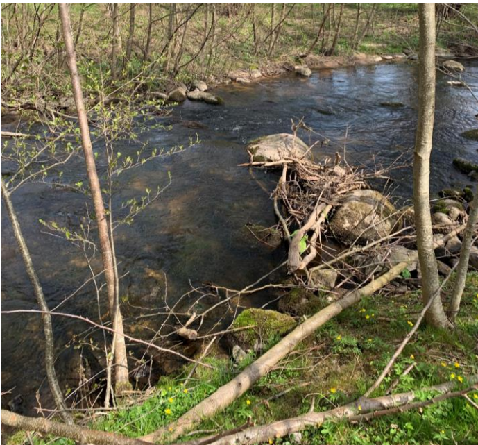
Figure 42. Upper bend of the fishway
