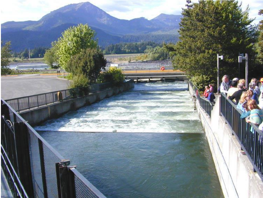
Figure 2. Pool and weir fishway at Bonneville dam on the Columbia River, USA.
