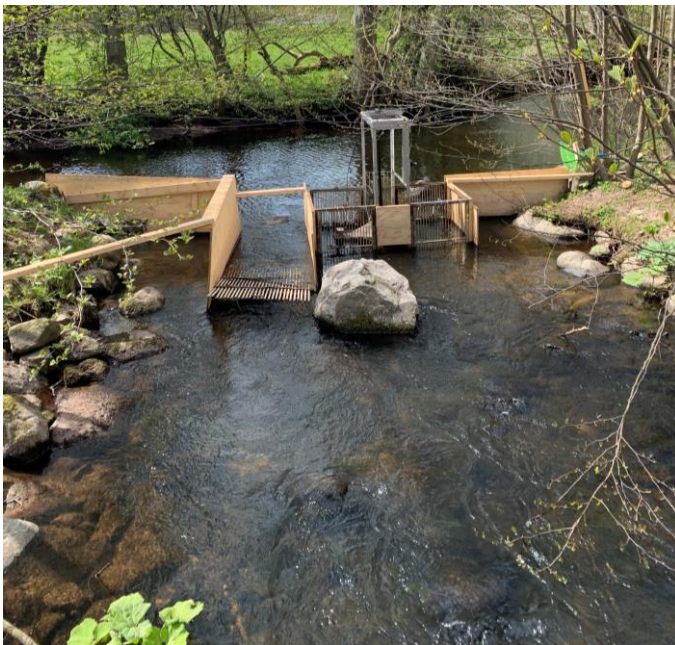
Figure 40. Upstream exit of the fishway with installed fishcounter
