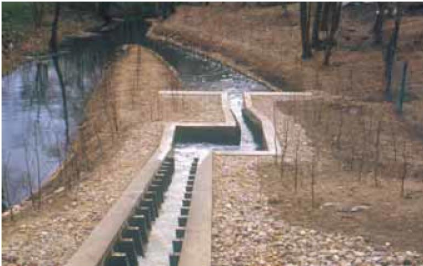
Figure 1. Denil fishway, Gillmitzer mill, Brandenburg, Germany (DVWK, 2002)
