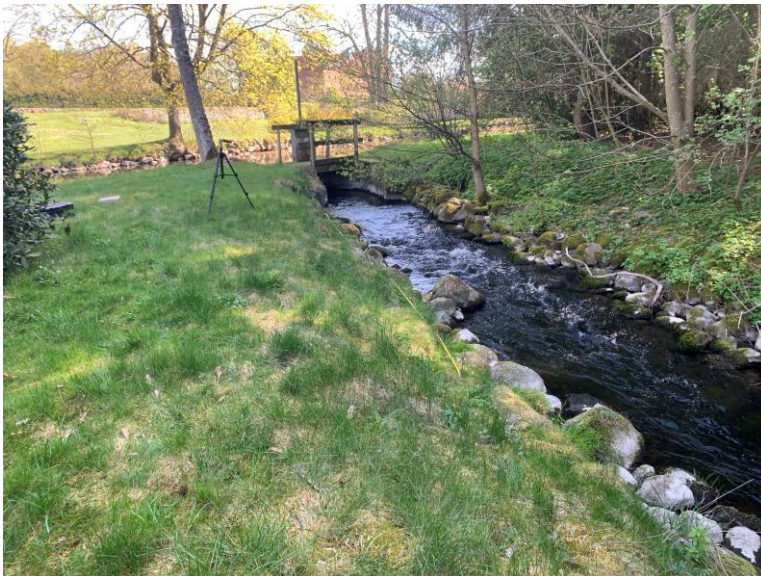
Figure 11. Upstream exit in concrete and upper most part of fishway.
