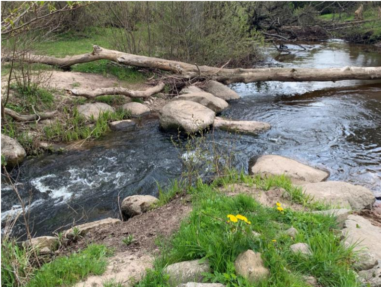
Figure 46. Downstream exit of the fishway
