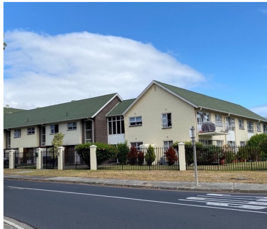
Figure 7.8 Two-storey houses for apartments in Pinelands.
