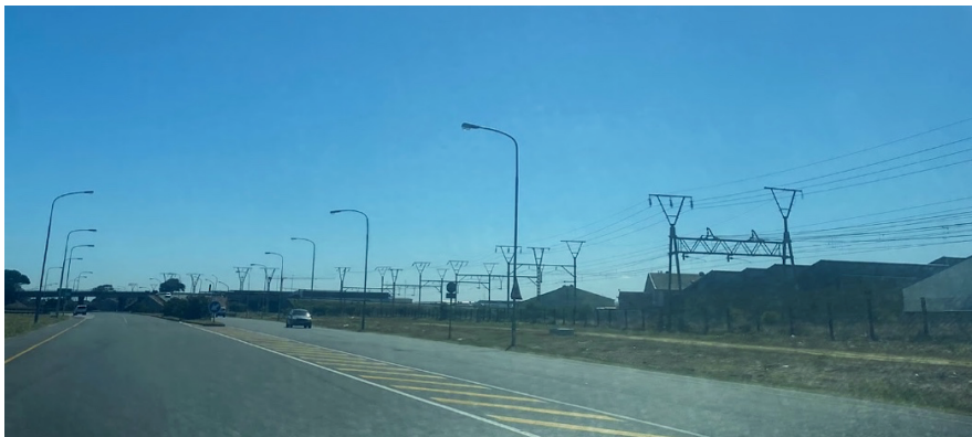
Figure 7.1 The railway and the highway are a barrier dividing Pinelands from the areas in its surrounding.
