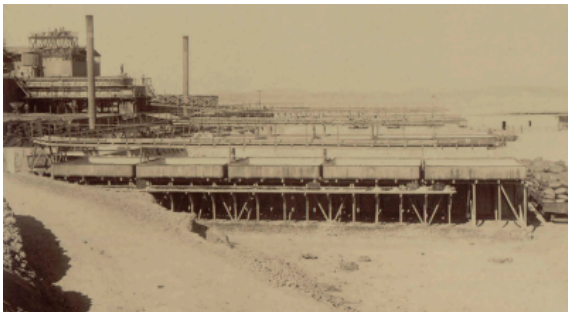
Leaching tanks at Democracia's Office
