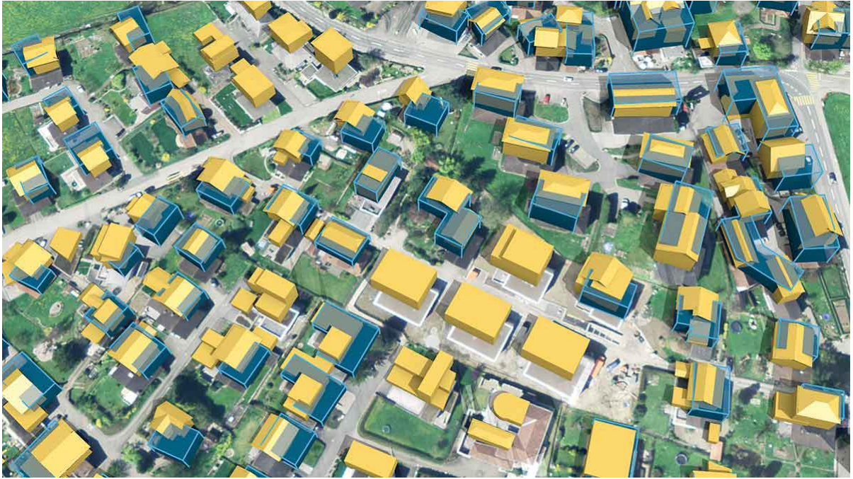
Figure 2.3: The illustration shows two datasets in different LoDs overlaid on an orthophoto (LoD1 – blue and LoD2 – yellow). The data is of the same area but with different accuracy and completeness due to being produced in separate campaigns. The data and the image is from Biljecki et al. (2018).
