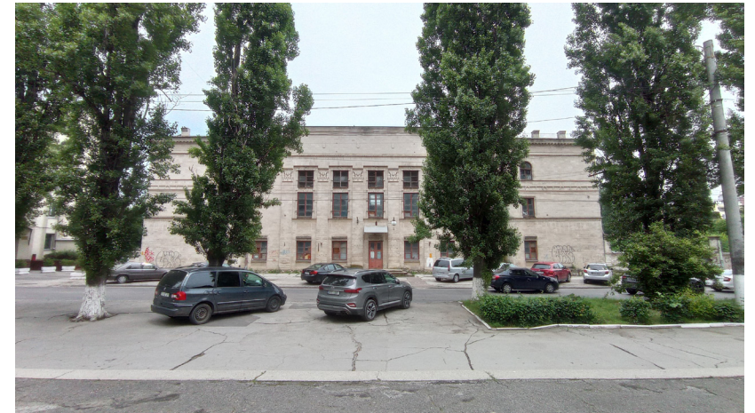
administration building of the Stadium, 2021. author photo
