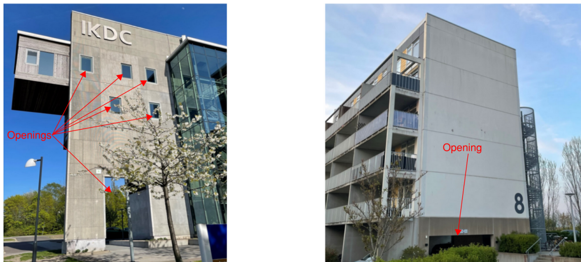
Figure 3.1: Two buildings that are stabilised with shear walls. Photos taken by Erik Bolin in Lund.
