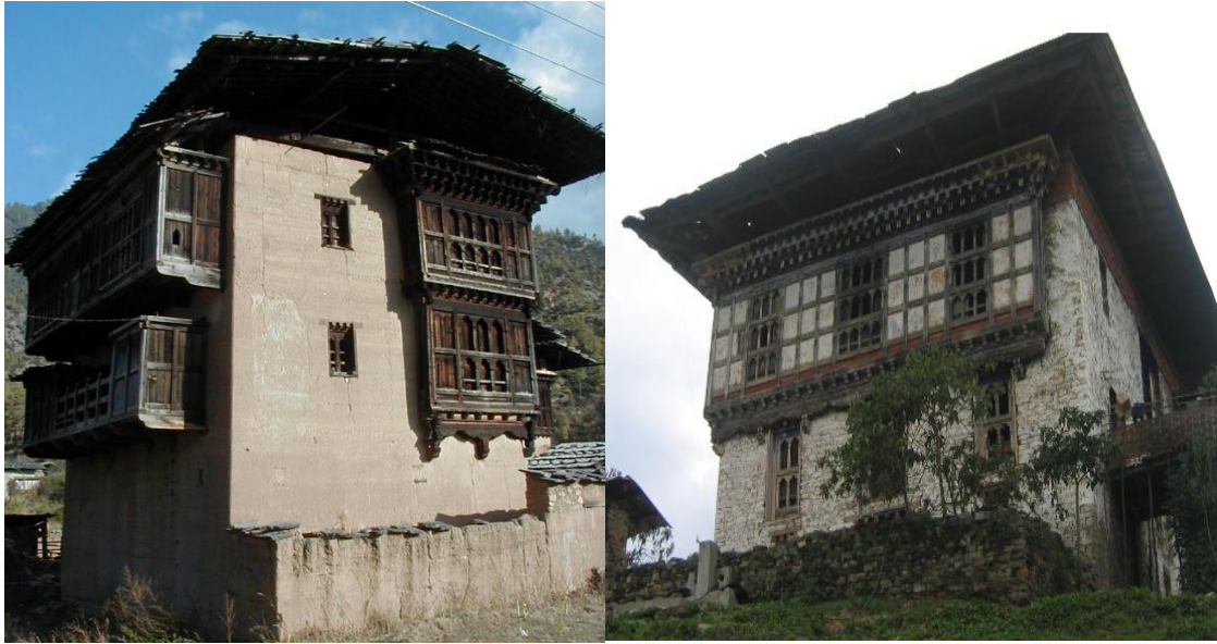
Figure 2.2: Traditional rammed earth and stone-wall buildings (MoWHS, 2014).
