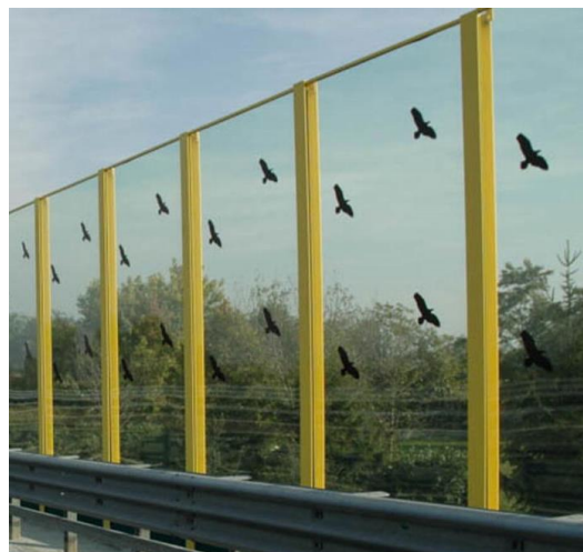
Figure 2.1 Hawks painted on the glass to scare birds off and prevents them from flying into the glass, which also works as a signifier for people to communicate that there is glass there [16].
