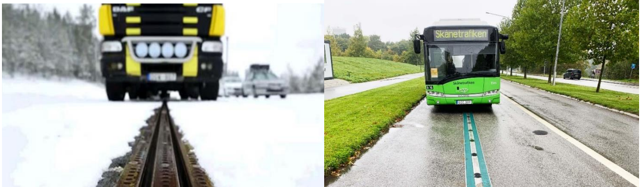
Figure 3. On the left: Elways' rail in the road (Kvaser 2017). On the right: Elonroad's rail on the road (Smart City Sweden 2020)
