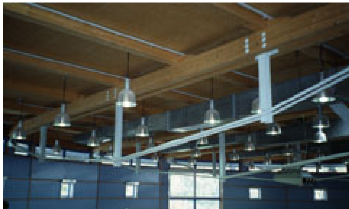
Figure 2.11: Cable-tensioned beam system. Träguiden [19].
