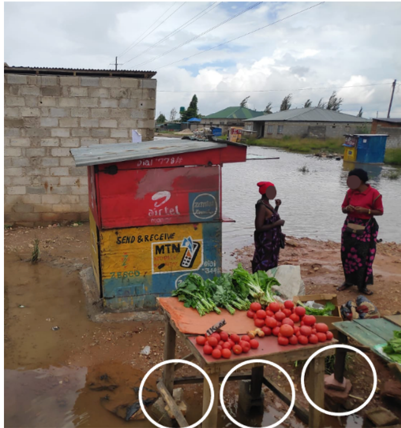
Figure 5-3 A market stall structure in Kanyama has been elevated above the water level with rocks.
