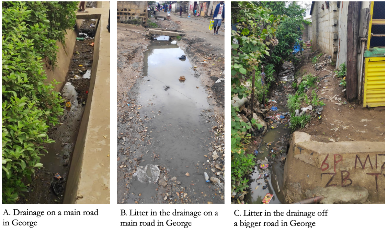
Figure 5-4 Drainage systems in Kanyama and George compounds
