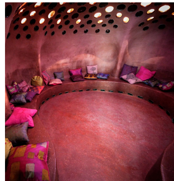
Omicron Monolith by Anna Heringer and Martin Rauch, 2014, Klaus, Austria. Earth walls shaped by hand, reinforced with geotextile webbing and clay vessels.
