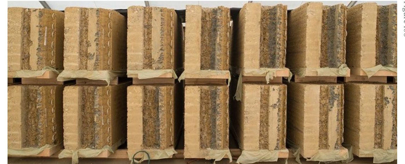
The insulation technique behind Alnatura Campus can be described as insulation material sandwiched in between the rammed earth structure. The structure was completed in 2019.
