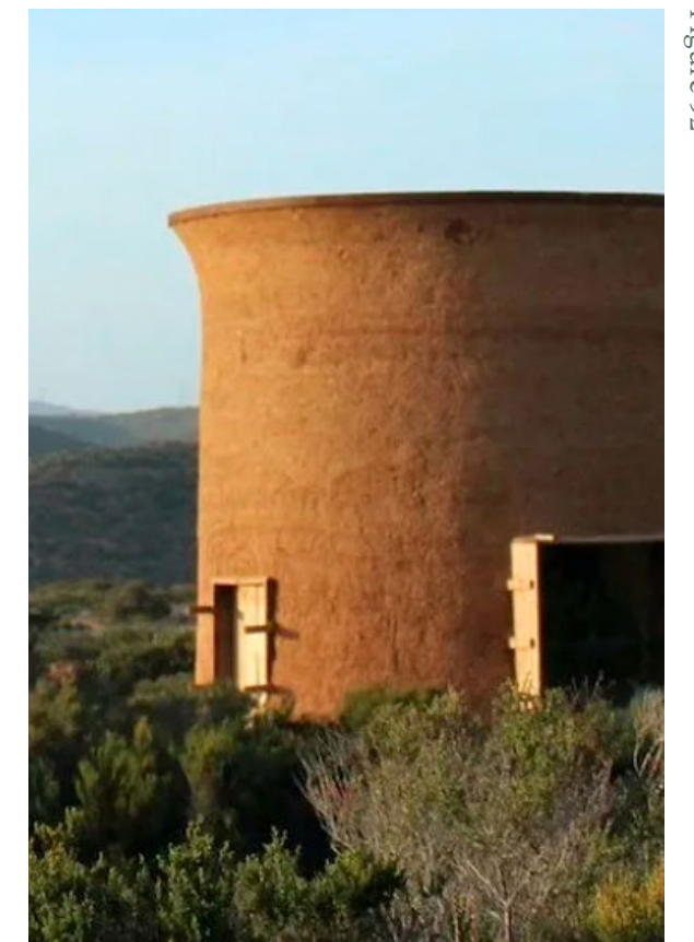
Galeria 2 Hijas, California by Cla Clá is entirely built out of cob. It was completed in 2021.
