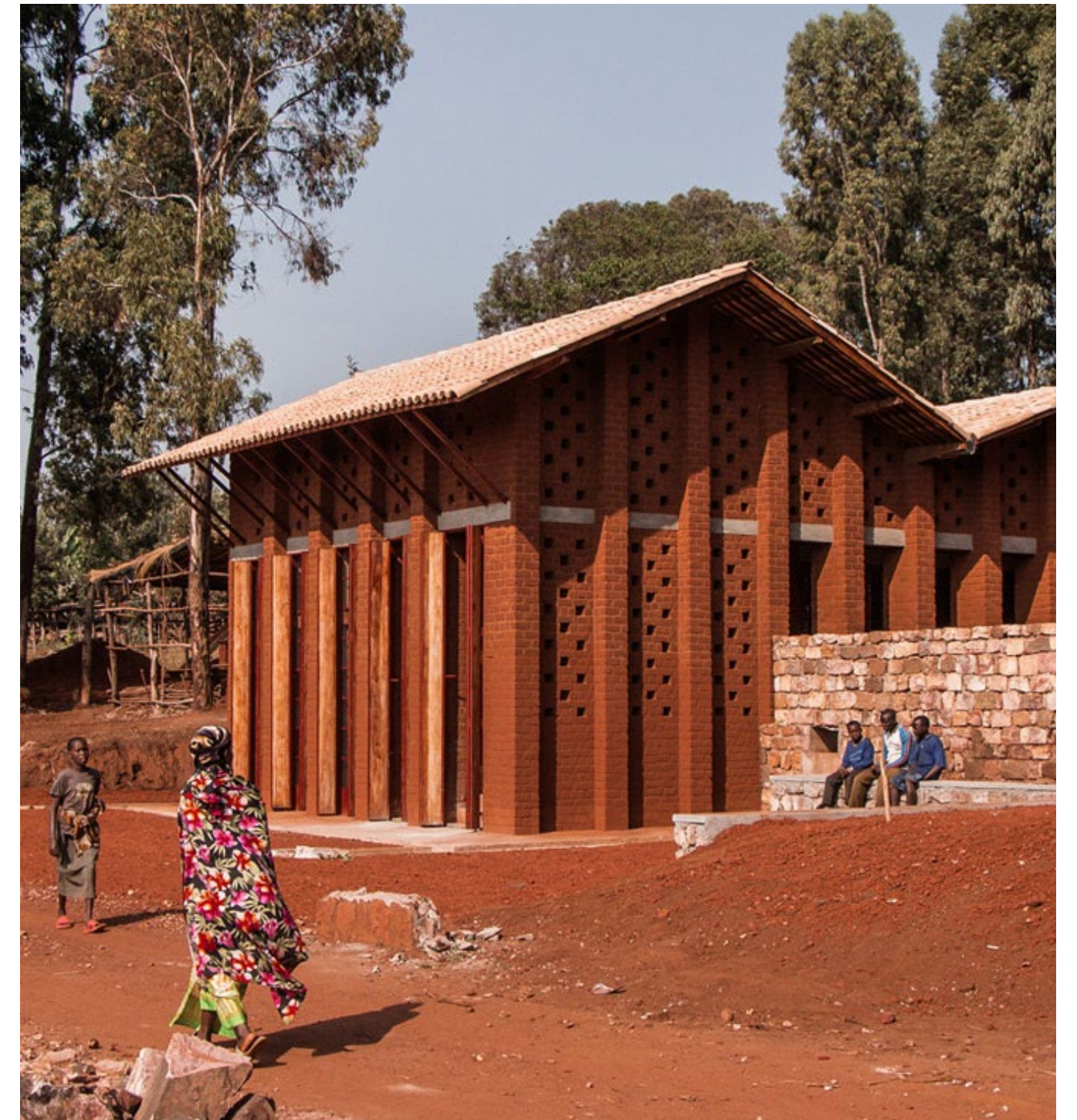
The materiality of the library is easy to read in this well-composed design. The ring-beam speaks of the load-bearing system and the use of perforated walls provides a compelling light-play.
