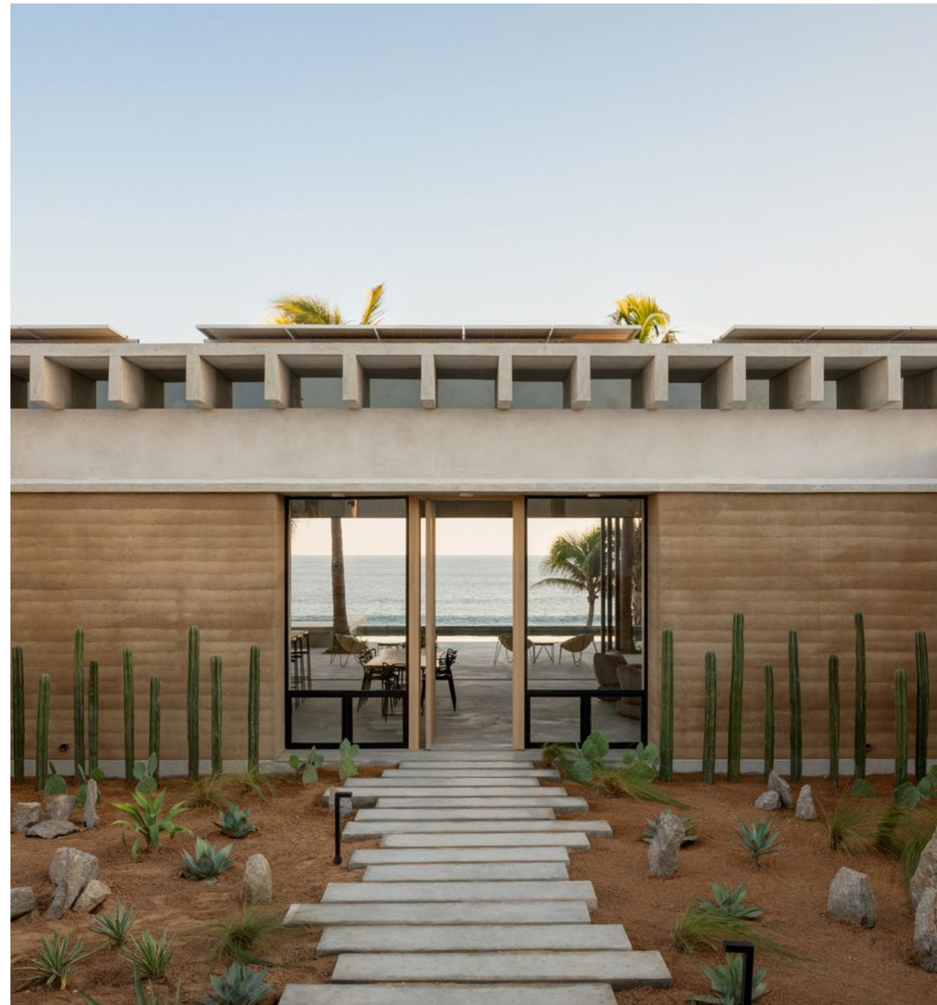
Casa Sal in Mexico by RIMA Design Group in 2020. The residential house is made out of rammed earth and cement.
