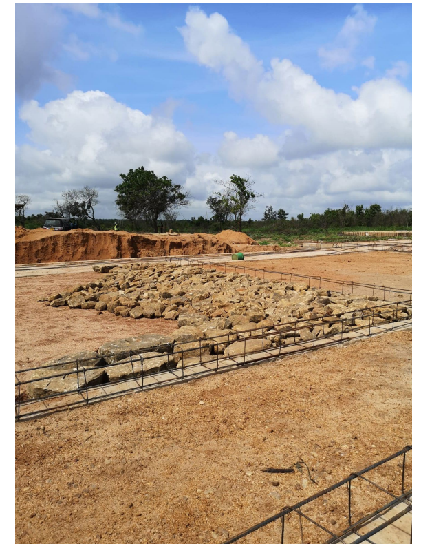
Figure 65: The rubble foundation. Each stone block is placed by hand.
