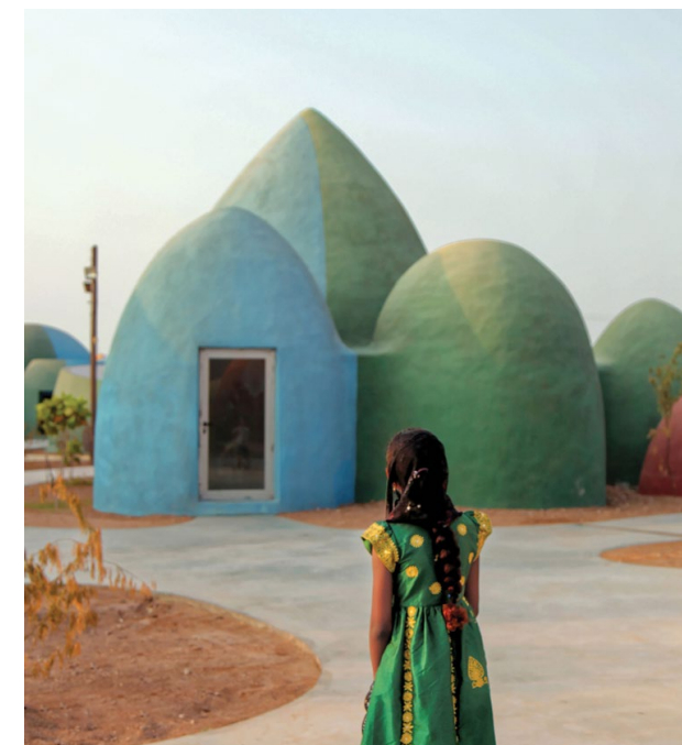
The Majara Village by Zav Architects features 200 pointed and rounded domes constructed out of plastered sandbags. Since 2020 it offers a creative and joyful environment for both locals and visitors of Hormuz, Iran.
