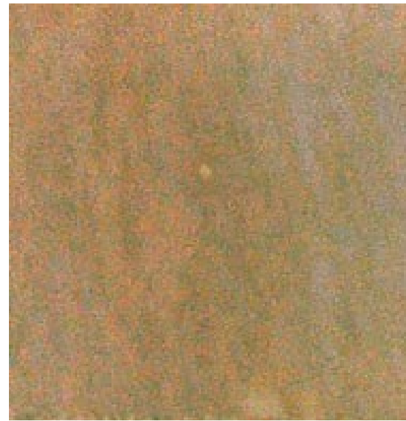
Manually tamped earth floor, polished by hand with stones, Gando Primary School by Keré Architects.
