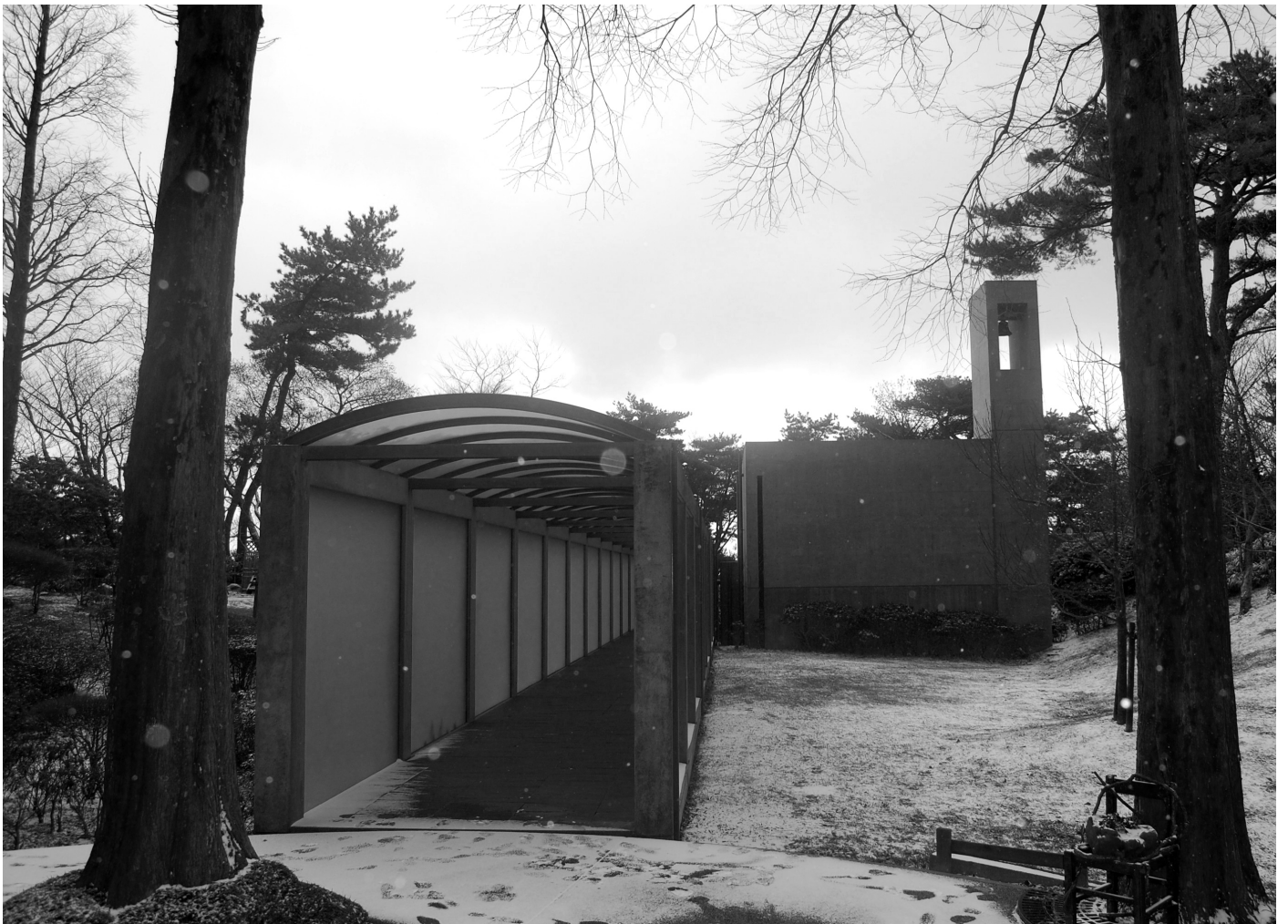
FIG. 18. START OF THE LONG "HALLWAY" AS AN ENTRENCE TO TADAO ANDOS CHAPEL VIEWED IN THE BACKGROUND (PHOTO BY: AZEVEDO FRANCA, 2006)
