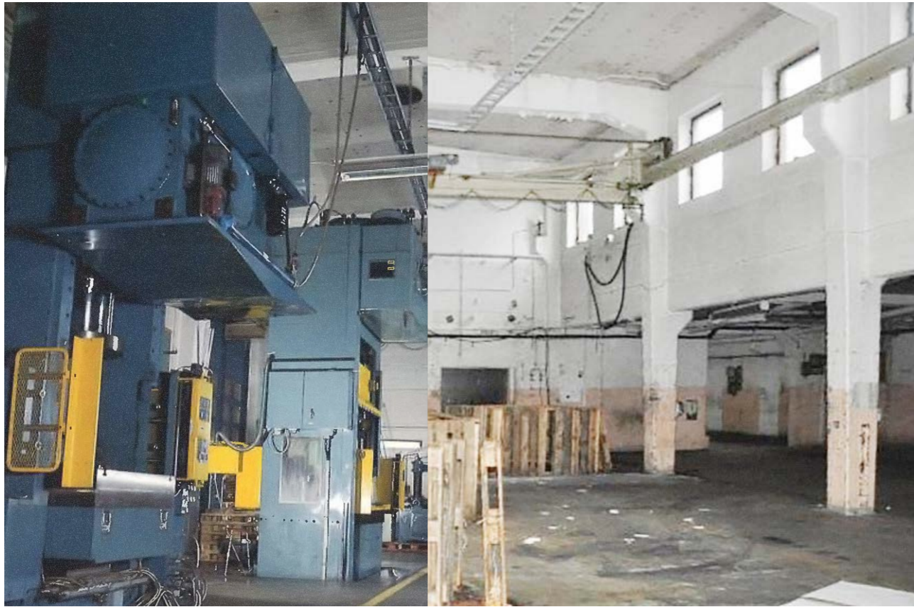
The machinehall in its past and current condition, photo from Ceba Steeltech & unknown (n.d.).
