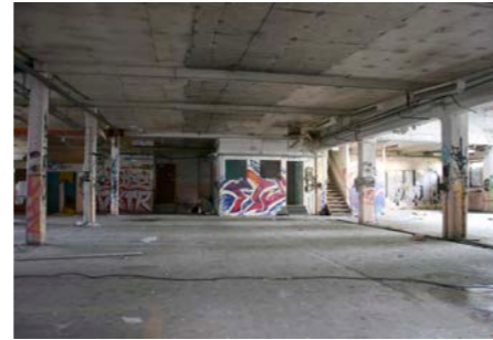
Disassembling the roof in the dark hall.
