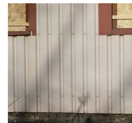
Facade plates from 1987 & window framing
