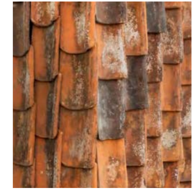
Facade of roof tiles (Nielsen, 2017)
