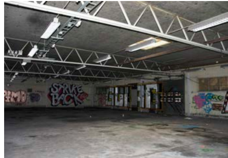
Disassembling truss structure from 1987.
