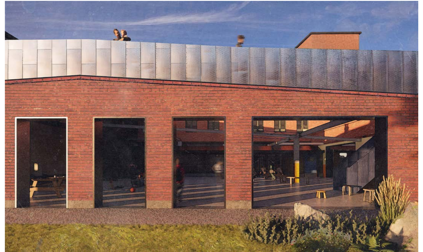
The former 'backside' as an opened up & inviting entrance to the courtyard.
