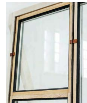
Frame system / Example of attachment by Vandkunsten architects (Nielsen, 2017)
