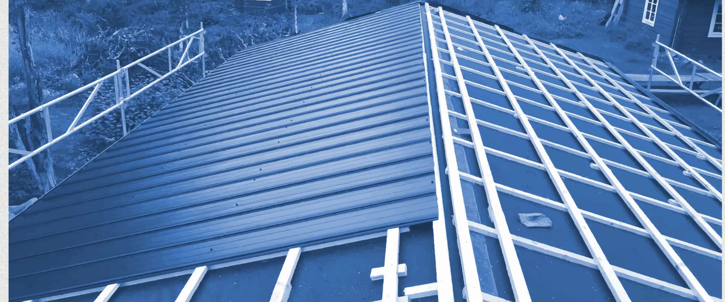
L's engineer boyfriend E, client H and her cousins J & P are currently on a coffee break before continuing to nail the steel roof in place.
