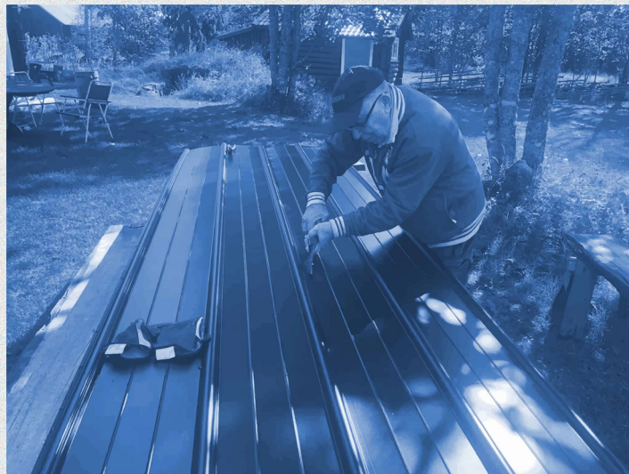
E's tinsmith grandfather B, 86 years old, cutting & bending the steel sheets to preferred size.
