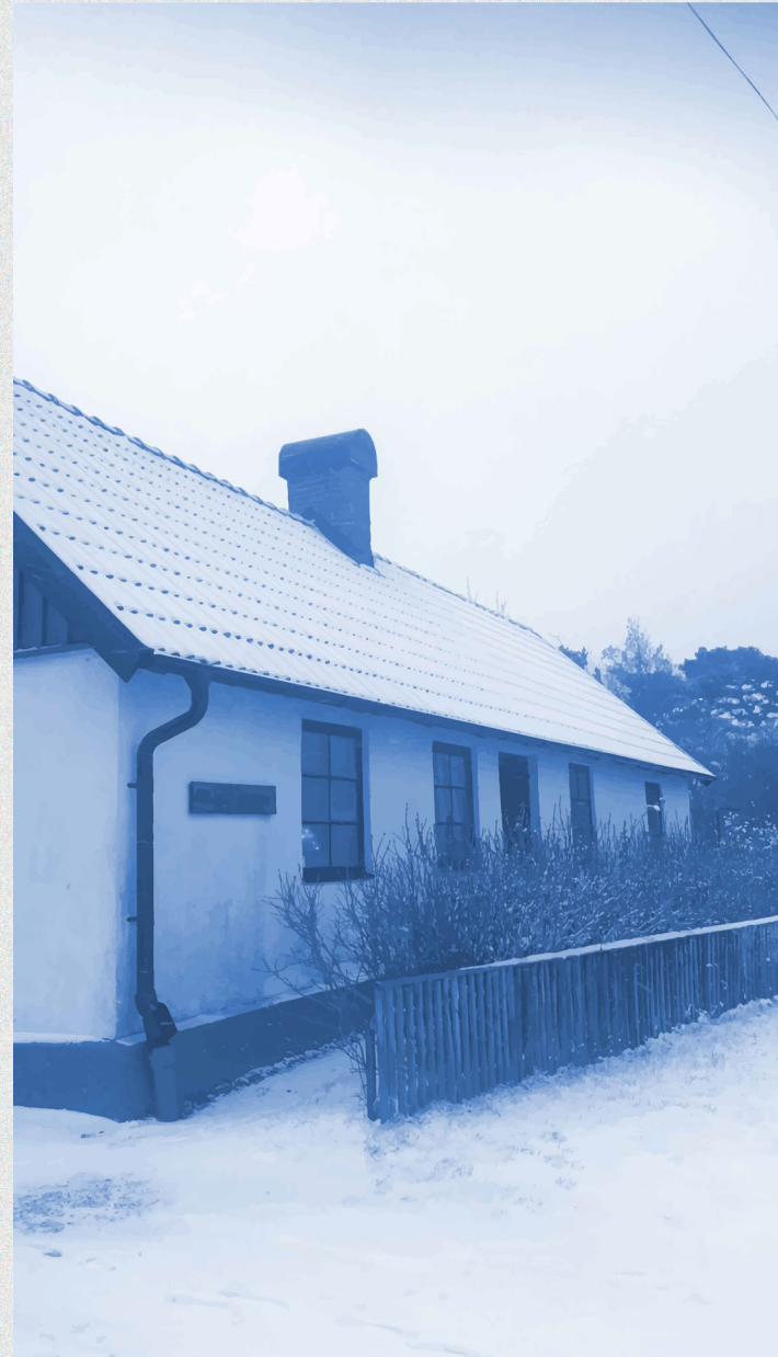
The east facade of the main building is facing the small gravel street & the open sea. The exterior was redone in lime plaster in the 1960's. A bit of the original wood cladding remains.
