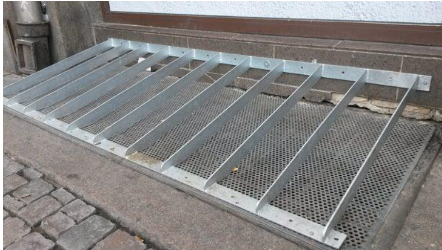
Figure 8: Slanting bars over a heating vent (Scheibye, 2017).
