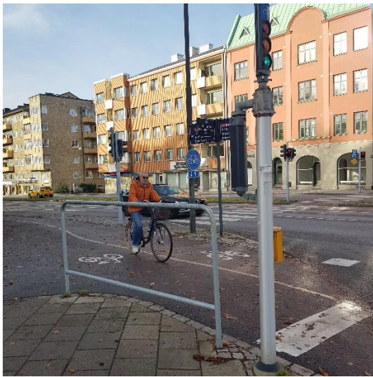
Image 1. Stop rails at traffic light
