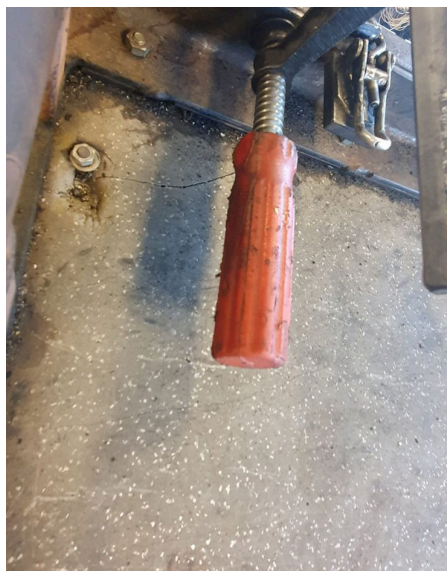
Figure 35: Crack above corner.
