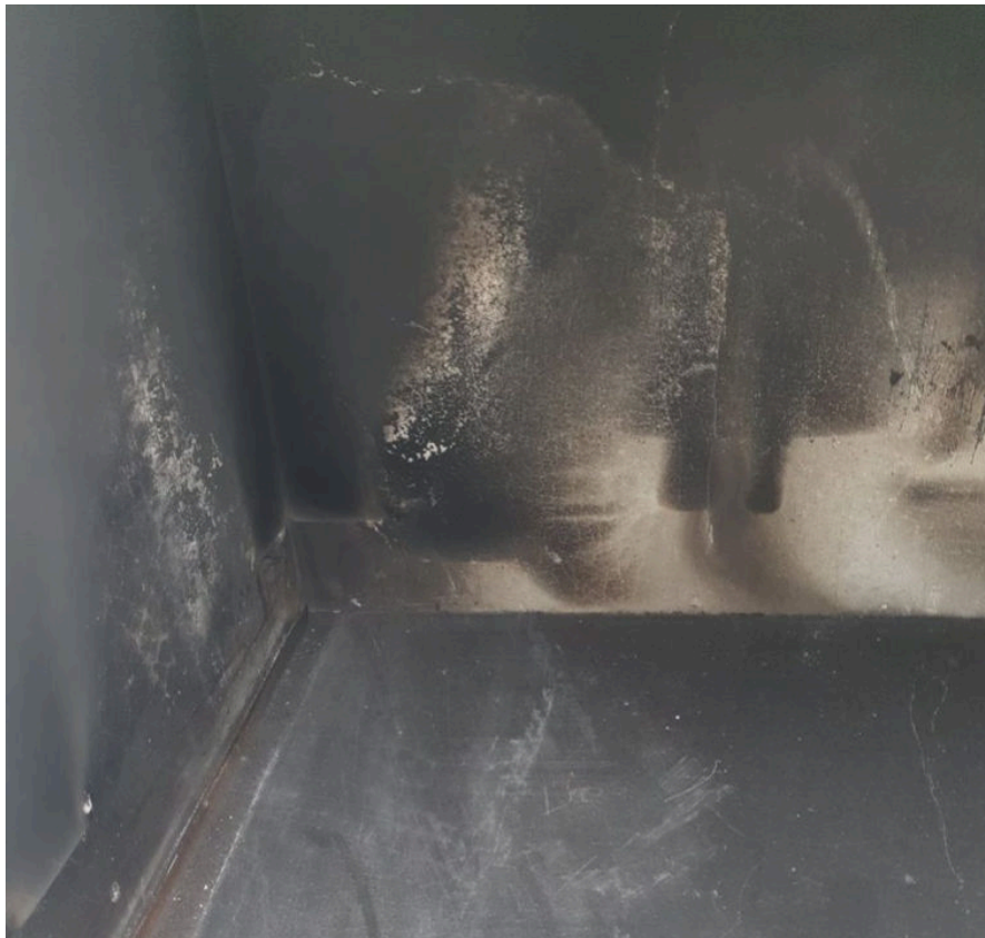
Figure 39: Crack inside the room.
