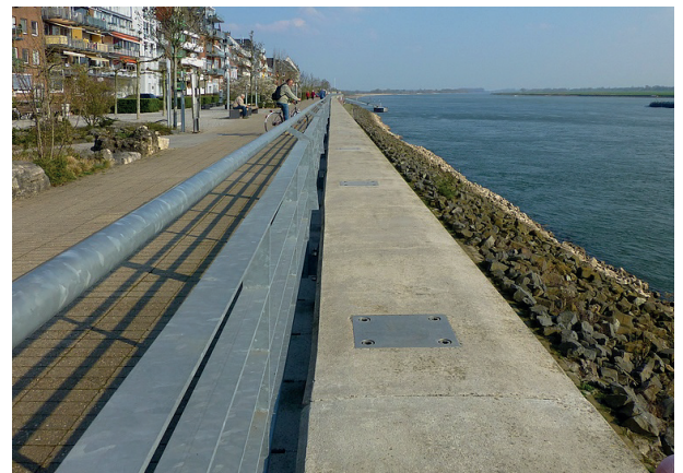
The flood wall can be elevated
