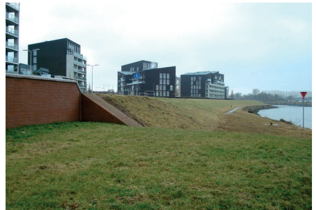
The flood wall can be elevated
