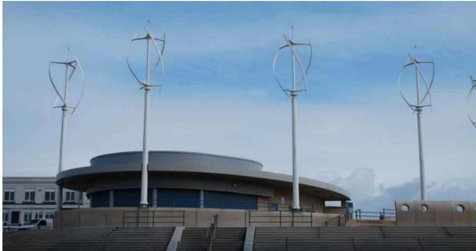
Figure 7. Photograph - QR6 Turbines on site. (Quiet Revolution, 2020). (Reproduced with permission from Quiet Revolution)
