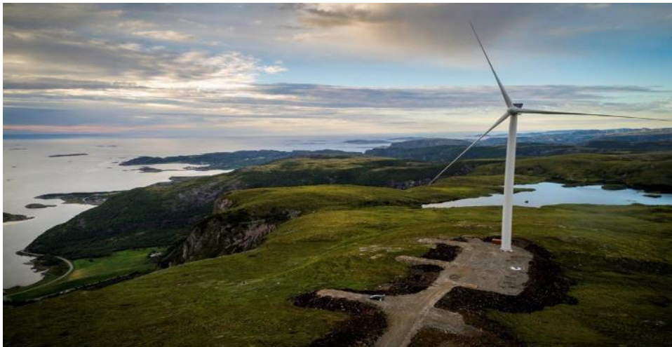
Figure 6. Photograph - Roan Wind farm
