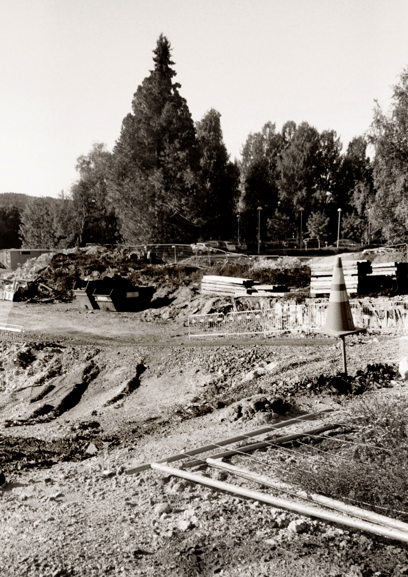
1. Image by the author in the site of the bridge construction.
