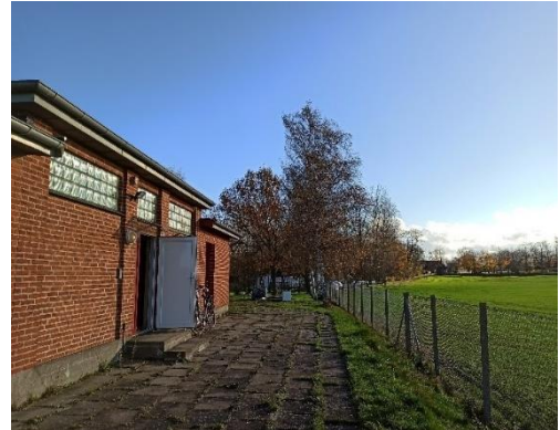
Figure 14. Waterworks at Lille Skensved.
