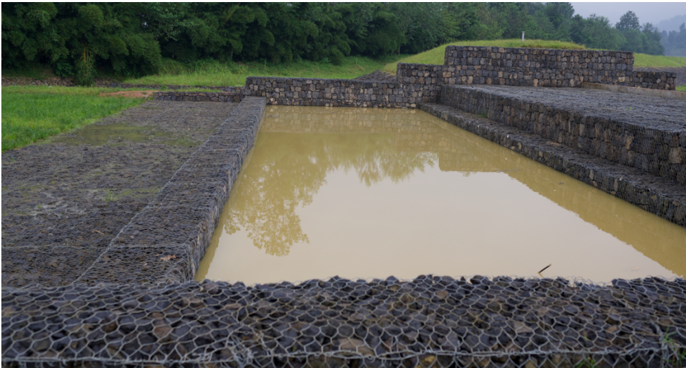
Figure 4-4 Outlet at Sebeya lateral retention dike.
