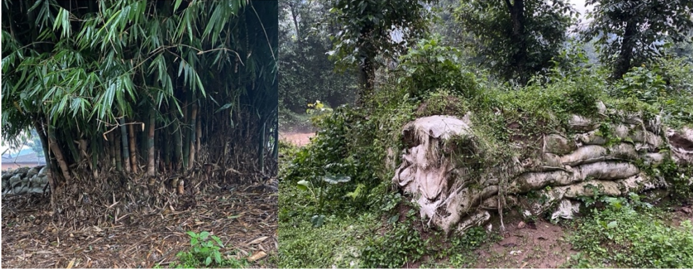
Figure 4-5 Bamboo and sandbags along the Sebeya River.
