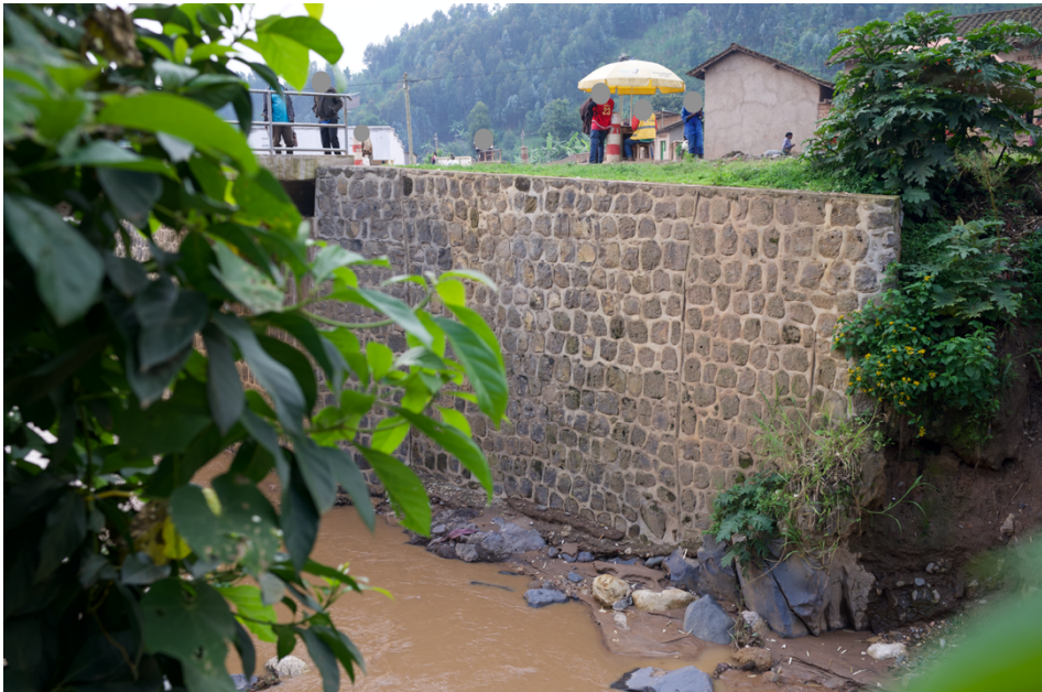
Figure A-5 Karambo retaining wall, downstream Karambo station.
