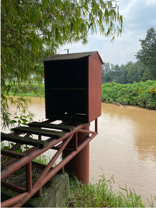
Figure 4-16 Decommissioned station at Gisenyi.
