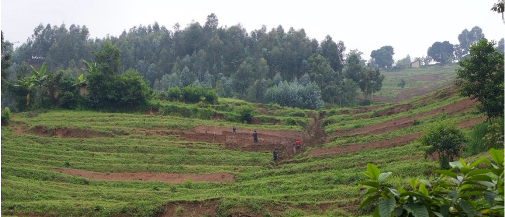
Figure 4-6 Terrace construction by Sebeya River.
