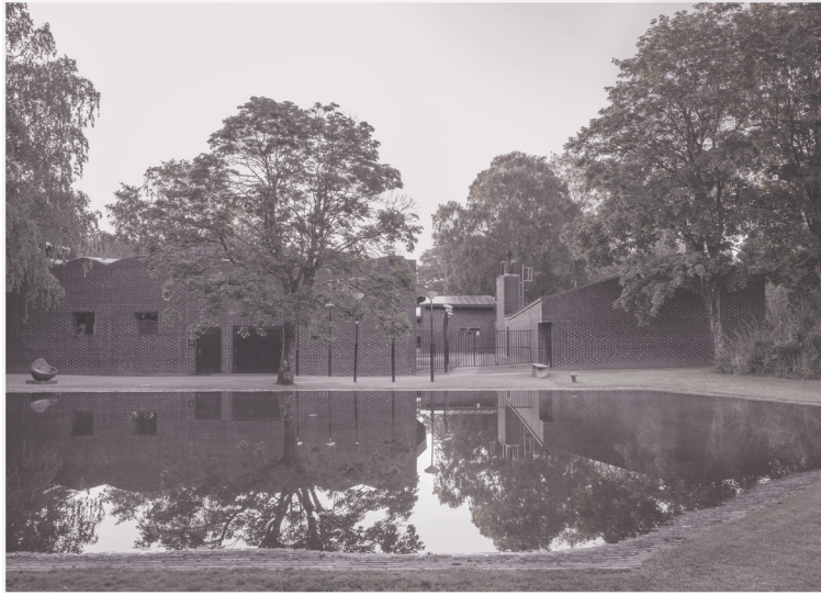
Figure 13: St Peters Church behind Klippan lake, Klippan, Sweden 2018. (Source: Architectural Reveiw,2018:Online)
