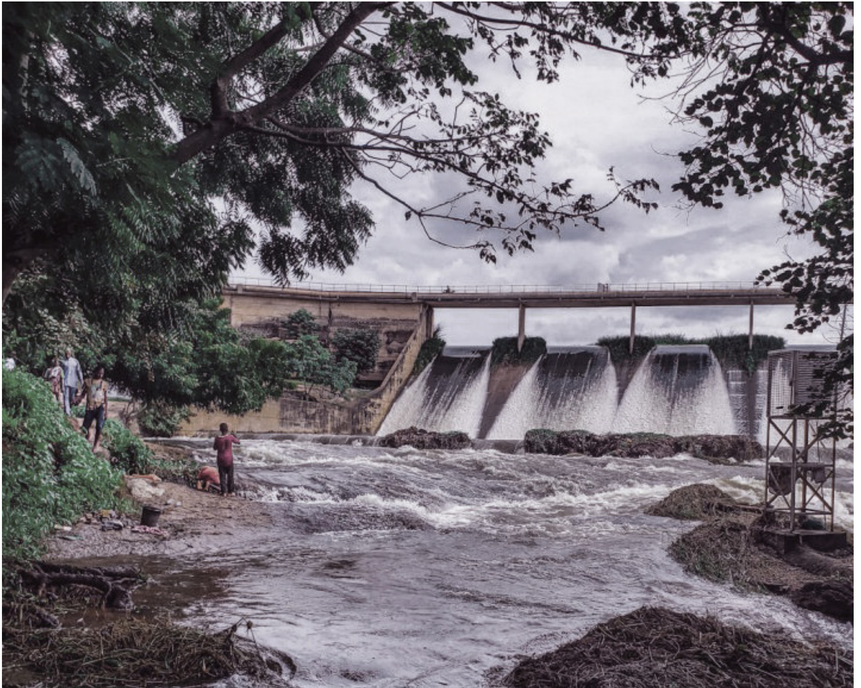
Figure 27: Asa dam, Illorin Nigeria 2022. (Source: Kwaraconnect,2022:Online)
