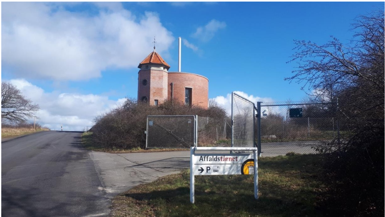
Figure 2: The Waste Tower at BOFA (own photo).
