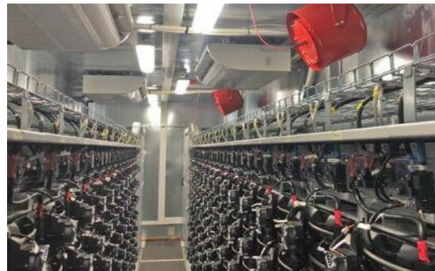
Figure 14 Aerosol system for battery room from RSL Fire [57].
