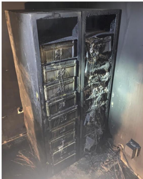
Figure 43 Aftermath of sprinkler water spray experiment. Left: Target Rack 1 and Right: TR Initiating Rack [116].
