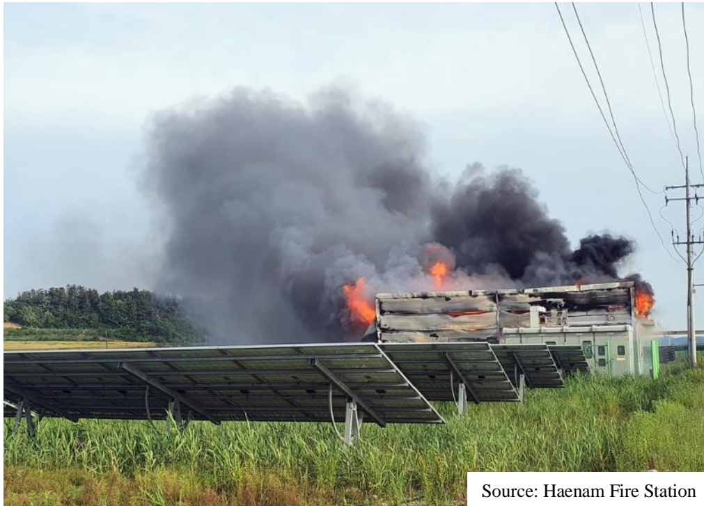
Figure 4 A fire broke out at a solar power BESS in South Jeollo, South Korea [23].
