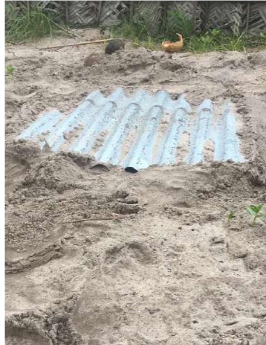
Figure 11: The aluminium plate covering the hole, with an air ventilation hole on the front side. The back side had the opposite holes open to allow the air to flow.
