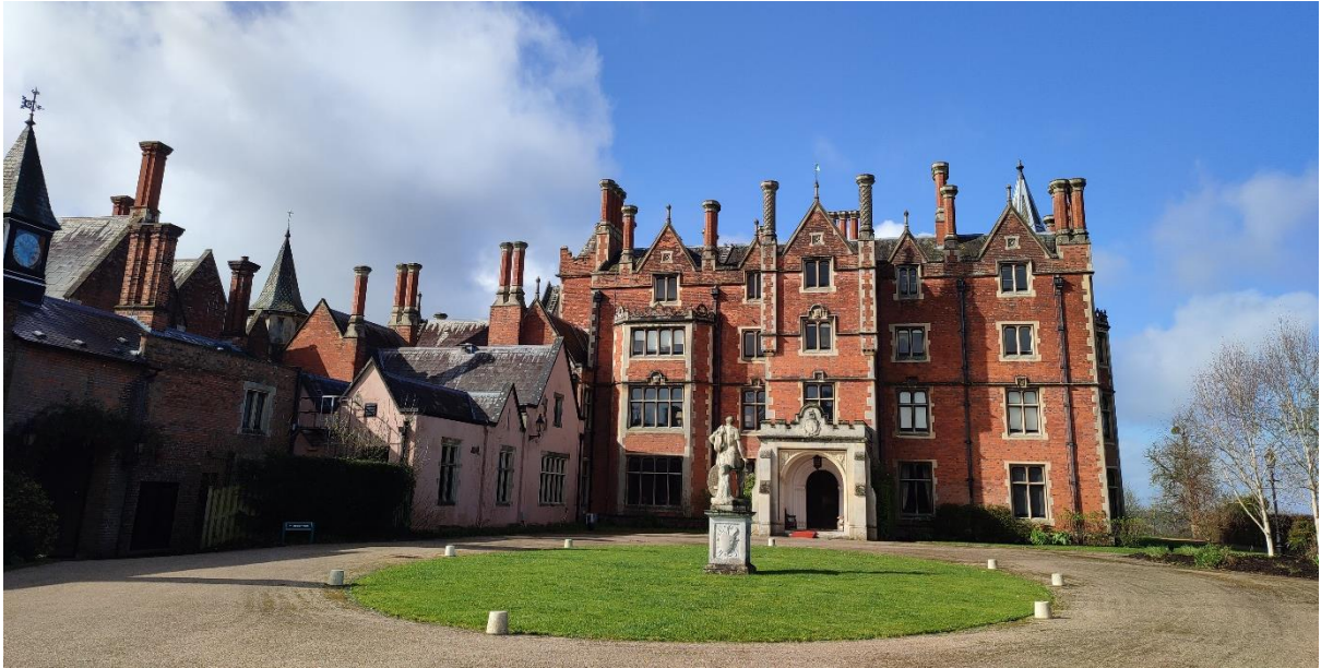
Figure 8: Taplow House, Taplow Court, UK. Photograph Taken with Mobile Phone by Author 22/03/2023.
