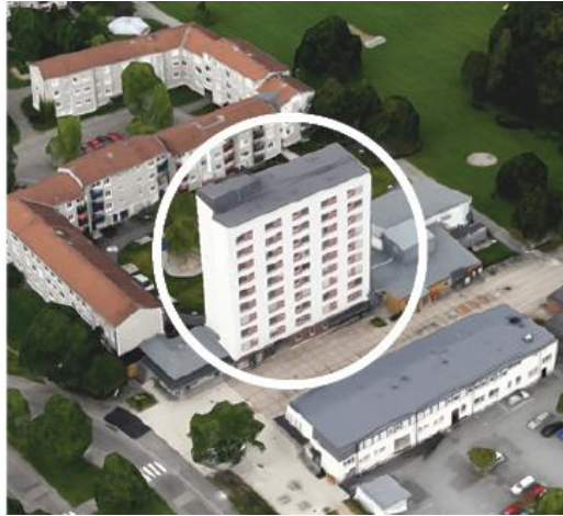
Figure 9 Aerial View of Building 22 (Baronbackarna B:5)
