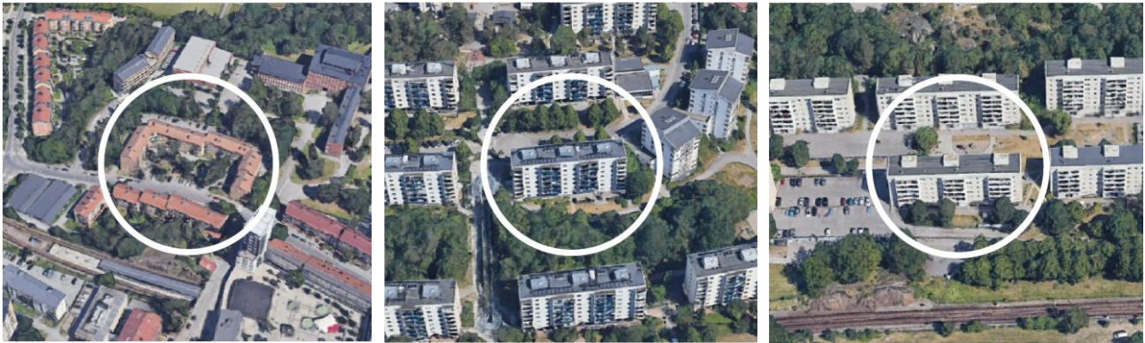
Figure 4 Aerial view of building 18 (left), 20 (middle), and 21(right)
