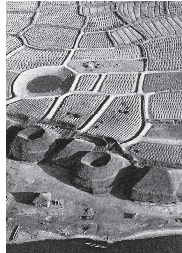
Impluvium houses in Senegal. Source: Holm and Kallehaug, 2015: 143 (photographer unknown). https://tmarch.com/fass
