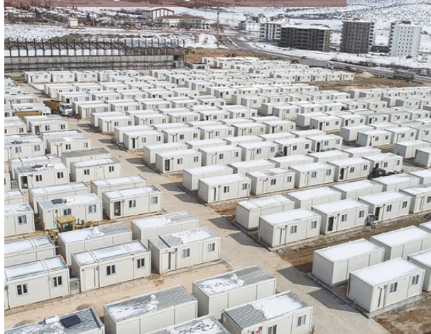
Fig.5: Temporary Housing in Elazığ, 2021
