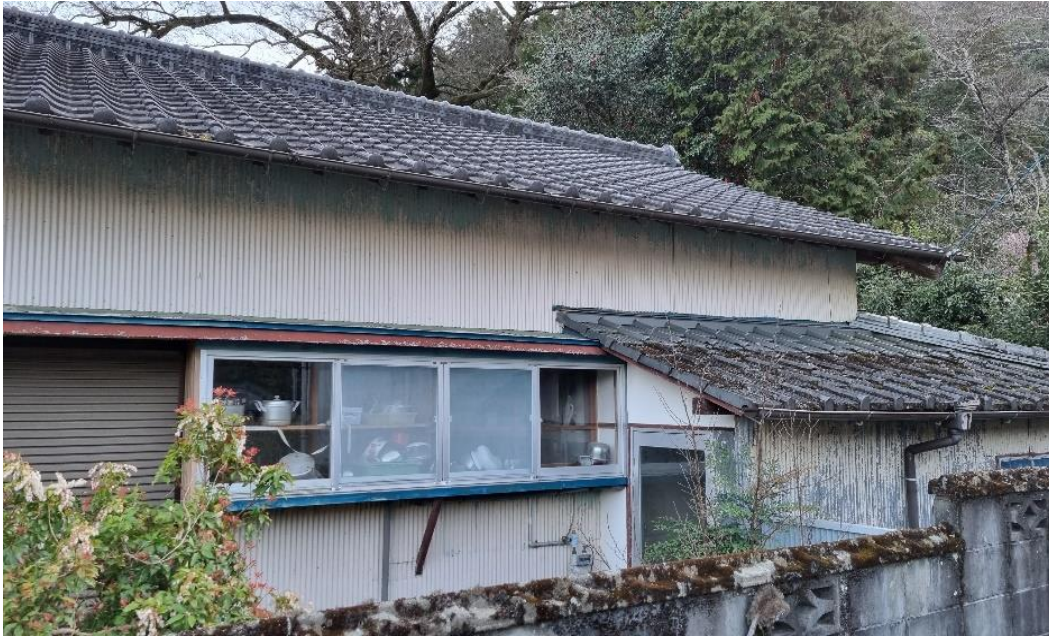
Figure 13. The akiya closest to Ken's house that he looks after. It is still full of things. Tosashi.
