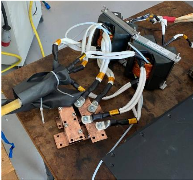
Figure 53 Paralleled capacitors and transformers and as the series to coil
