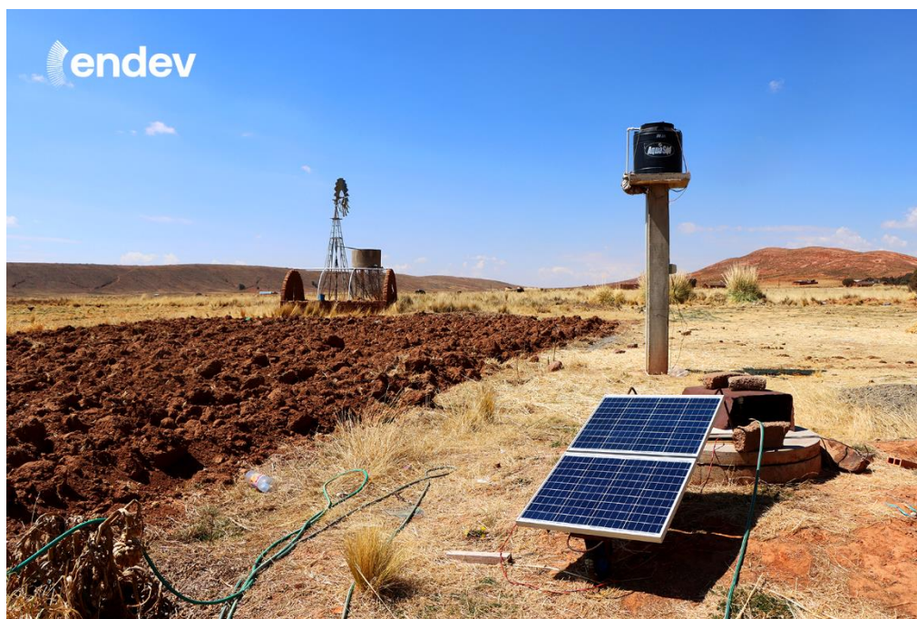
Figure 2-3. Solar water pump implemented by EnDev Source: EnDev Project Bolivia, GIZ
