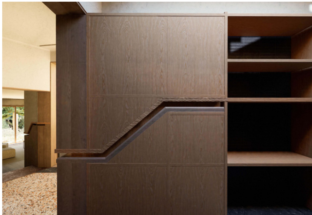
The guiding line that goes through the building becomes handles for the stairs, the handles are then integrated into a wardrobe.
