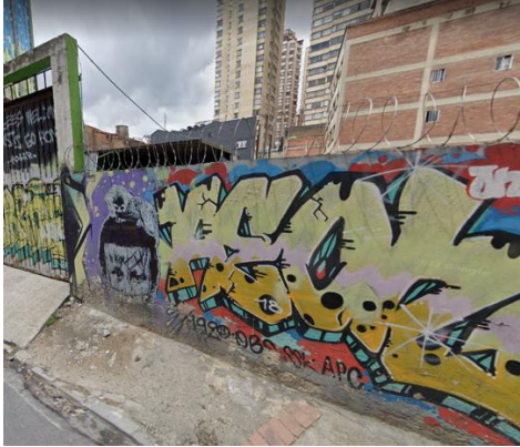
Figure 6.6. Example of wall with wires, protecting a parking lot (Google Maps, 2020)
