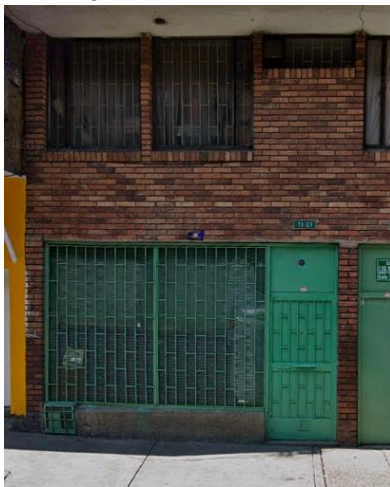
Figure 6.26. Example of bars on windows and doors in Las Nieves (Google Maps, 2020)
