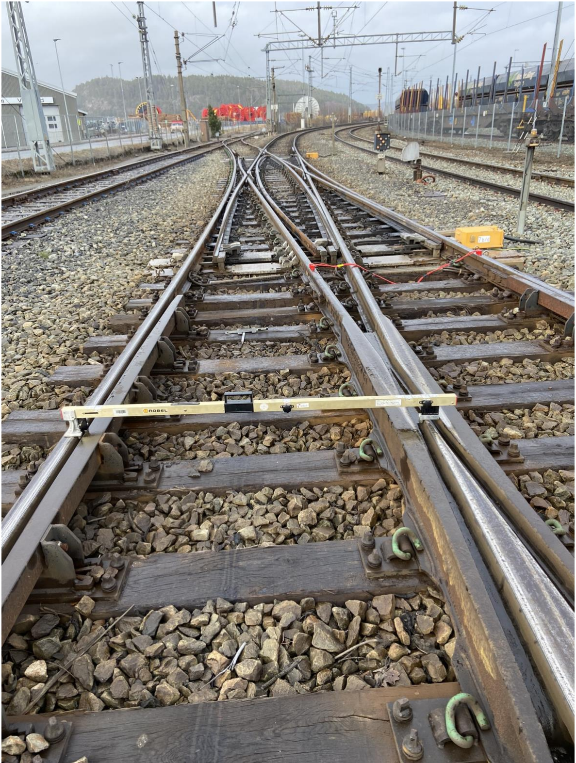
Figure 5, Crossing measurement during field study with spirit level
