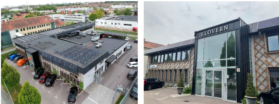
Fig.2: Aerial view of the building in study (left); Kabingatan 9, Malmö, Sweden. Photography by Sahit TM
