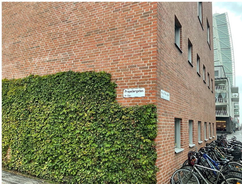
Fig.1: Example of an outdoor green wall in Malmö, Sweden; 2022. Photography by Sahit TM
