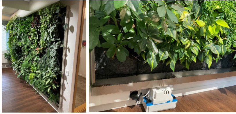
Fig.6: Detail of the metallic framework- outer protection structure (left), and draining duct at the bottom of the green wall. Photography by Sahit TM
