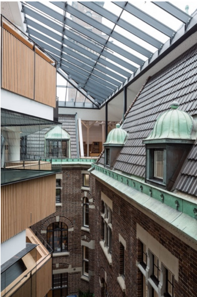
Figure 6: Interior of WMU, with historic roofline encased inside the new build addition on left.
